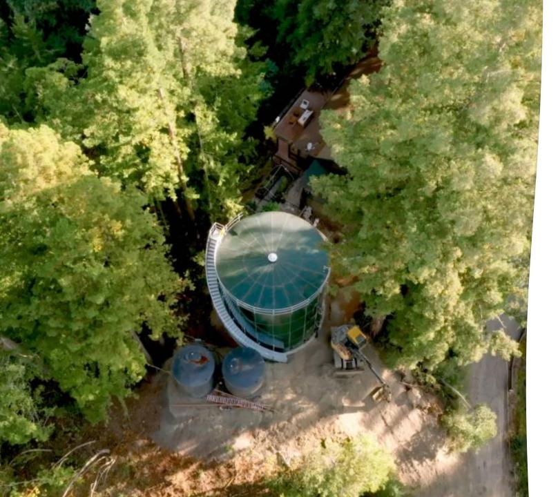
The project replaced an undersized redwood tank for a steel tank three times the size. The upgrade increased the amount of water available for customer use and firefighting purposes.
