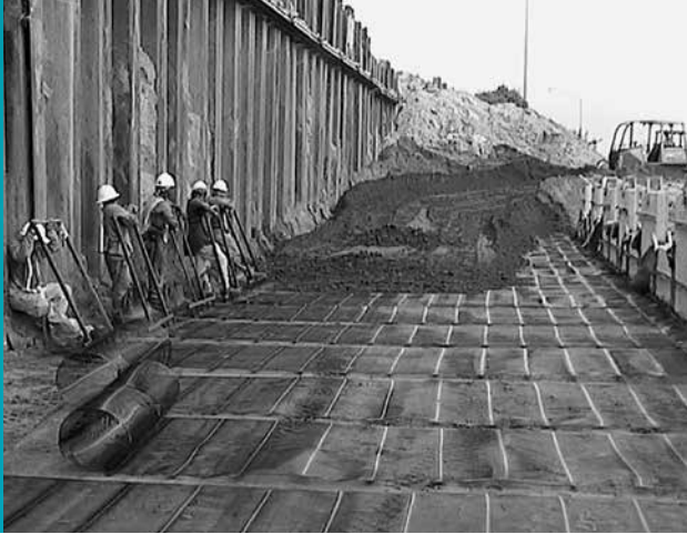
IMAGE Q: Geogrid tensioning and fill placement process.
