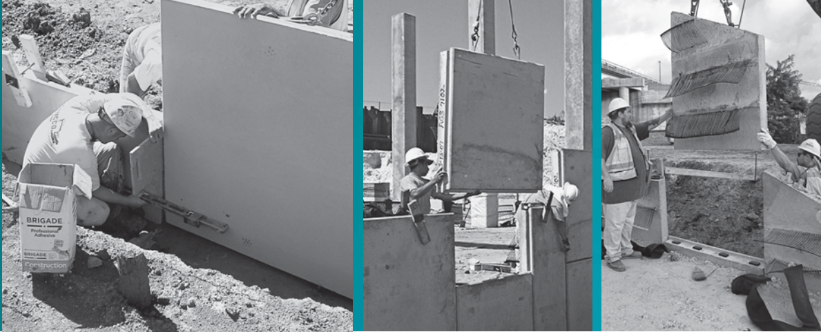
IMAGE J: Placement of 5 x 5 panels.
