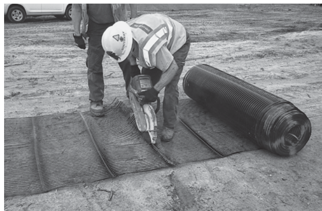
IMAGE D: Safe cutting of geogrid may be accomplished with a variety of cutting tools. Care should be taken to avoid cutting the transverse bar.
