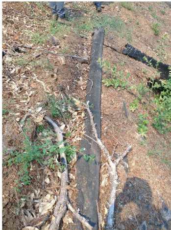
PICTURE #3 MELTED PIPE – 5 MILE
