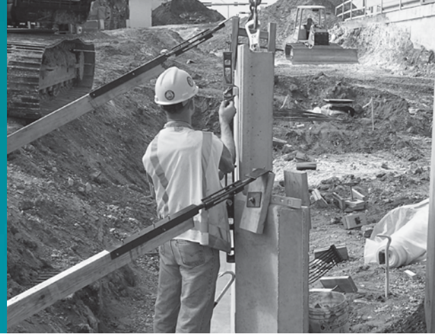
IMAGE I: Establishing batter of ARES® panels.
