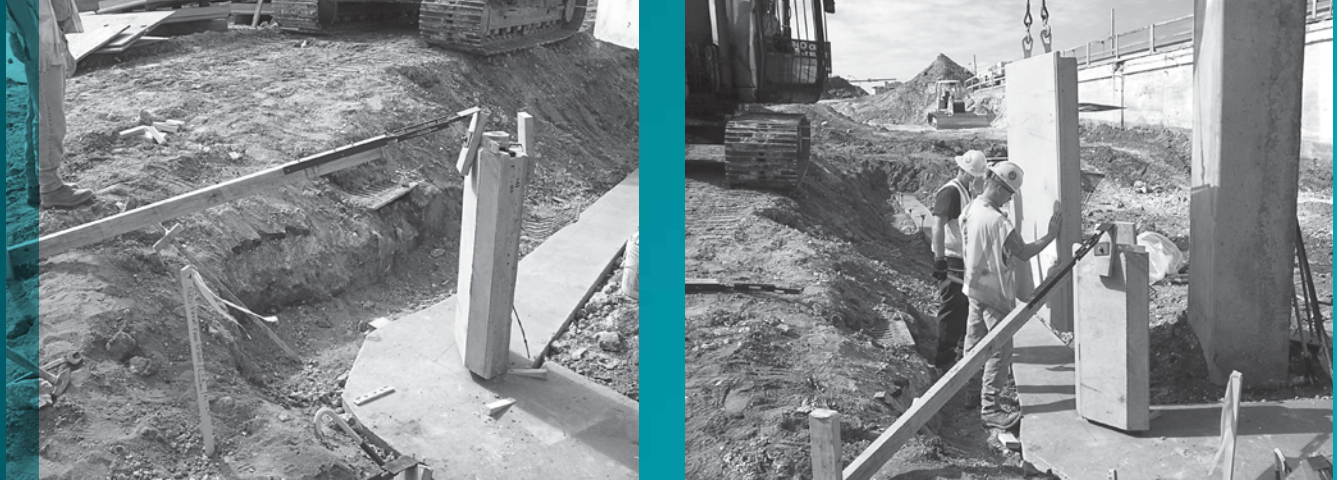
IMAGE E: Panel placement commonly begins at corner locations. Placement and bracing of concrete panels.
