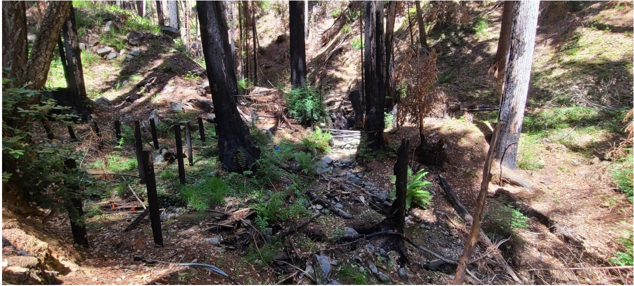
Photograph 4: Clear Creek #1 Crossing with Remains of Above Grade Crossing Structure
