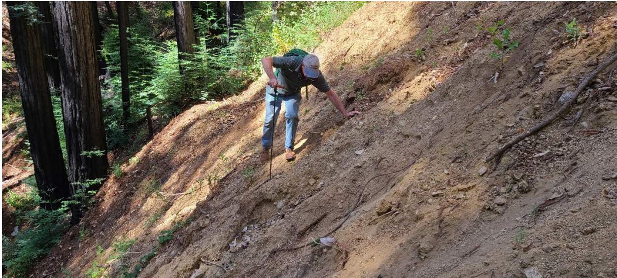
Photograph 3: Area of Extremely Steep Slopes where Cutbank Landsliding Impacted Existing Waterline Bench
