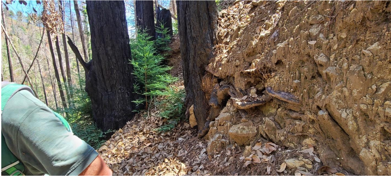
Photograph 8: Example of Extremely Steep Slopes, Unstable Conditions and Closely Spaced Trees along Existing Waterline Bench
