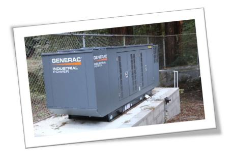
New Generator high enough to avoid water damage
