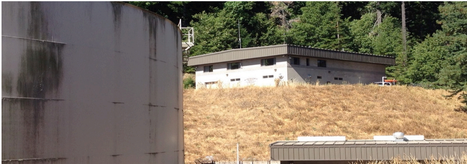
Lyon Treatment Plant
