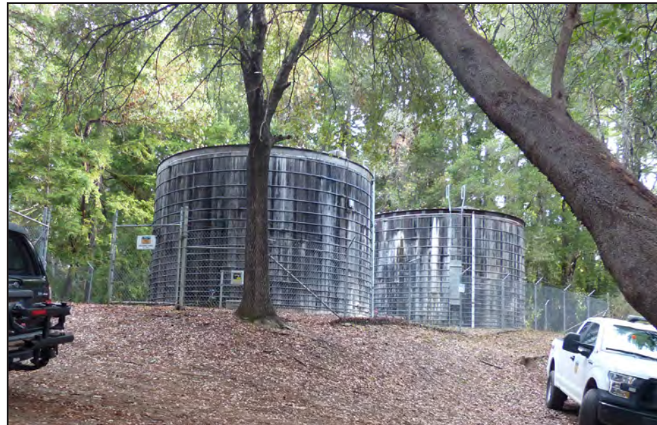
Photo 3: View of Madrone tank site looking north, showing the existing leaky redwood tanks.
