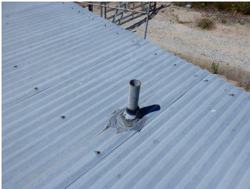
Photo 2-Roof penetration mastic
