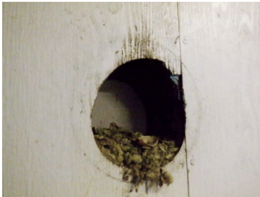
Photo 10-Wall paneling with fiberglass insulation
