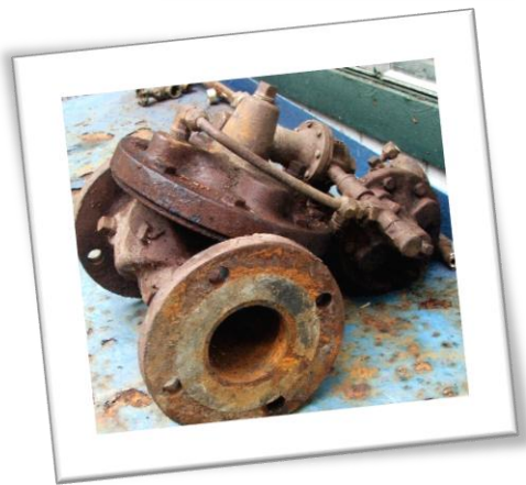
Used valve from PRV station
