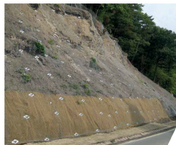
Above: SPIDER® on rock slopes The spiral rope made of three twisted, high-tensile steel wires is characterized by its high puncturing resistance. At the same time it is unobtrusive and can be tightly secured around protruding rock boulders.
