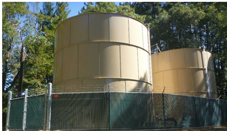
Madrone Site – Twin 75,000 gallon tanks, 26' Ø, 25' H
