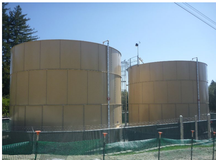
Lewis Site – Twin 114,000 gallon tanks, 32' Ø, 25' H
