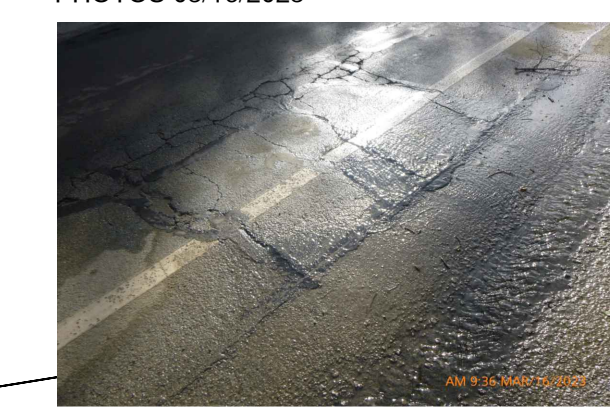
PARALLEL PG&E GAS TRENCH HIGH WATER TABLE PHOTOS 03/16/2023
