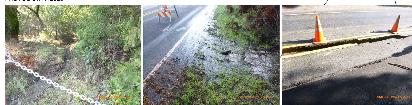
JANUARY STORM DAMAGE REPAIRED BY SANTA CRUZ COUNTY PUBLIC WORKS DEPARTMENT & GRANITEROCK PHOTOS 01/17/2023
