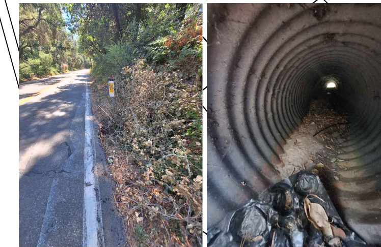
EXISTING CULVERT CONDITION PHOTOS 08/23/2023
