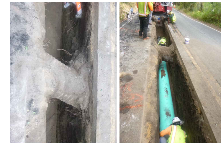
EXISTING CULVERT CONSTRUCTION PHOTOS 08/05/2022
