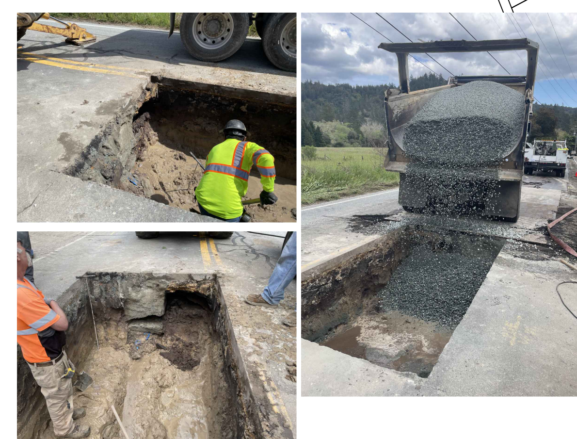
MARCH STORM DAMAGE REPAIRED BY SLVWD & ANDERSON PACIFIC PHOTOS 04/18/2023
