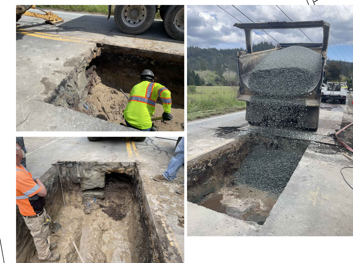
MARCH STORM DAMAGE REPAIRED BY SLVWD & ANDERSON PACIFIC PHOTOS 04/18/2023
