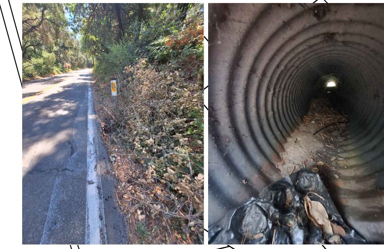
EXISTING CULVERT CONDITION PHOTOS 08/23/2023
