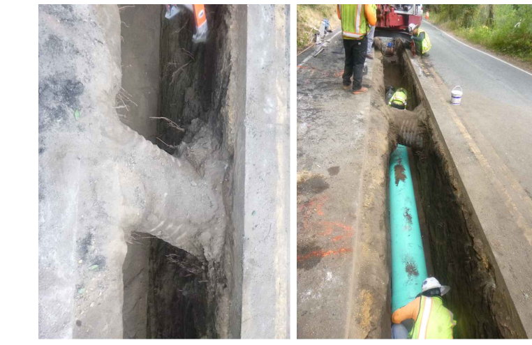
EXISTING CULVERT CONSTRUCTION PHOTOS 08/05/2022
