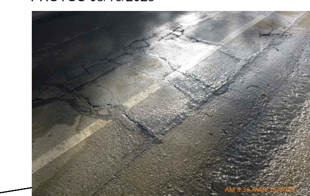
PARALLEL PG&E GAS TRENCH HIGH WATER TABLE PHOTOS 03/16/2023
