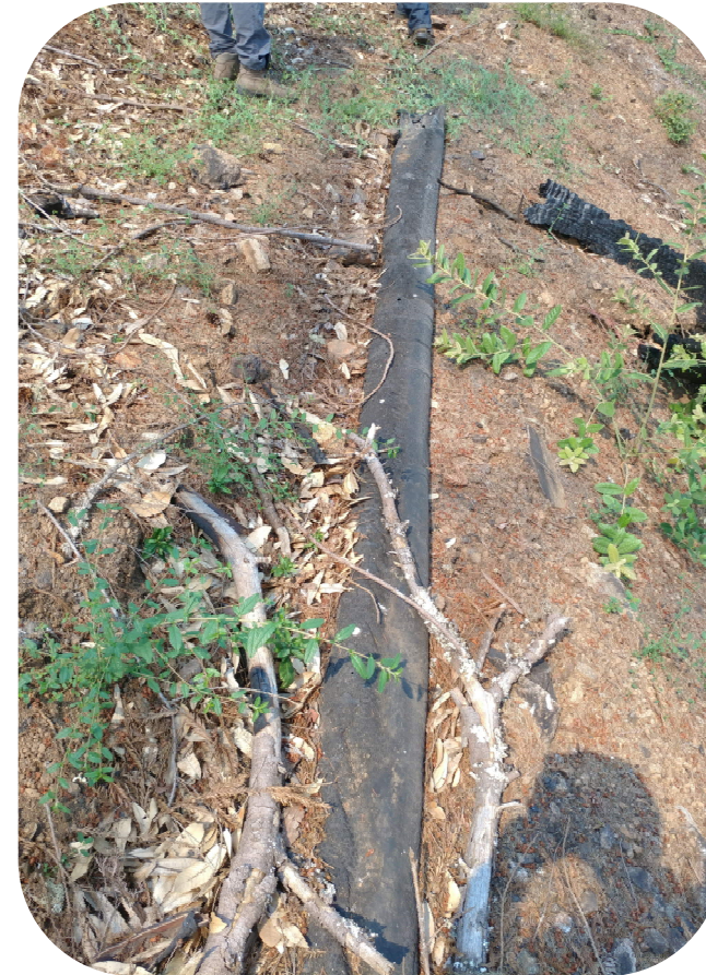
Irreparable pipe damage
