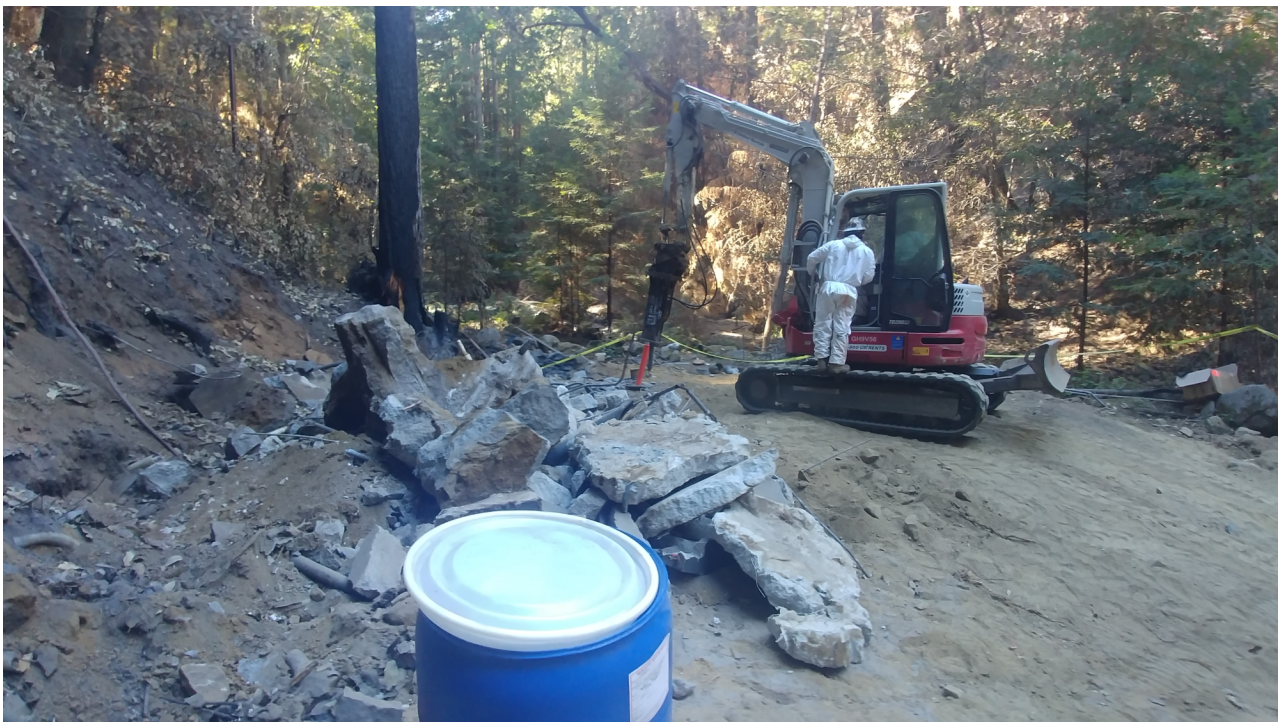
Figure 2: Removal of Hazardous Materials at Foreman Intake Pressure Break Structure
