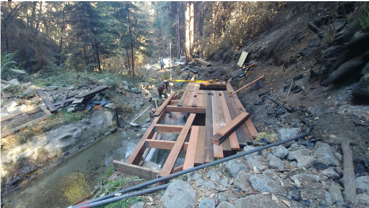
Figure 4: Construction of new intake structure cover at Foreman Intake
