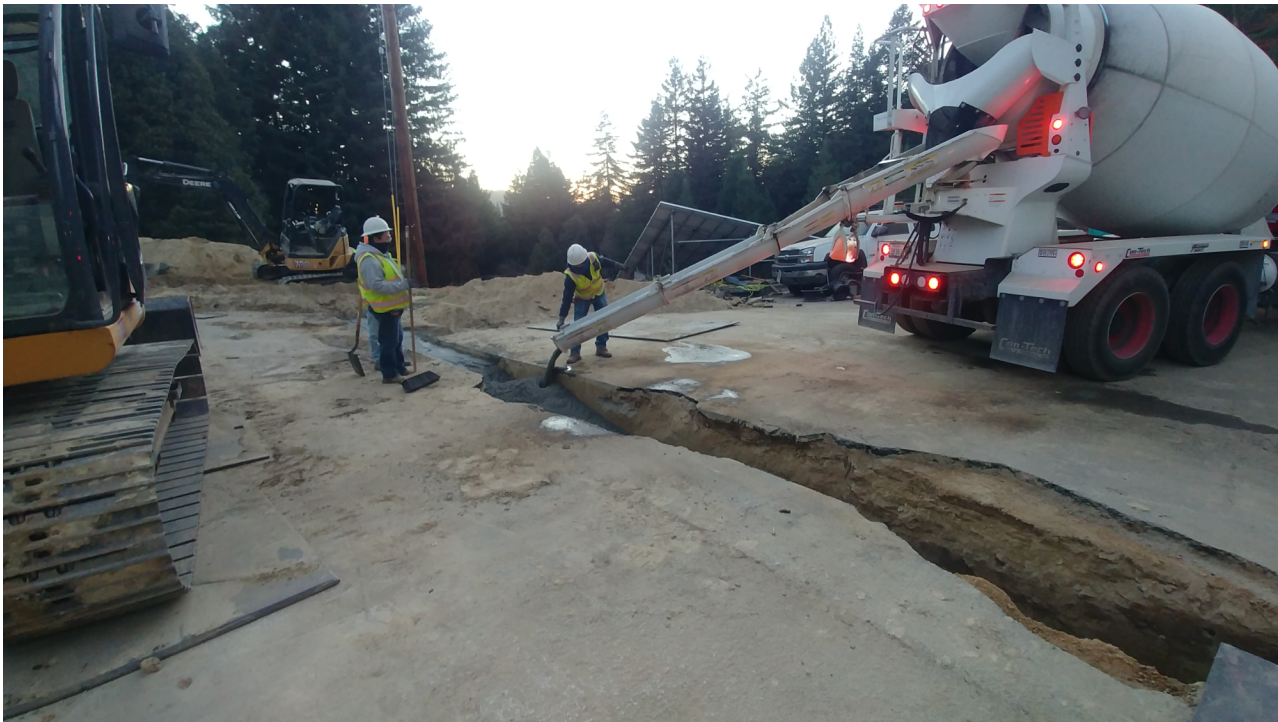
Figure 1: Slurry Backfill near Lyon Tank
