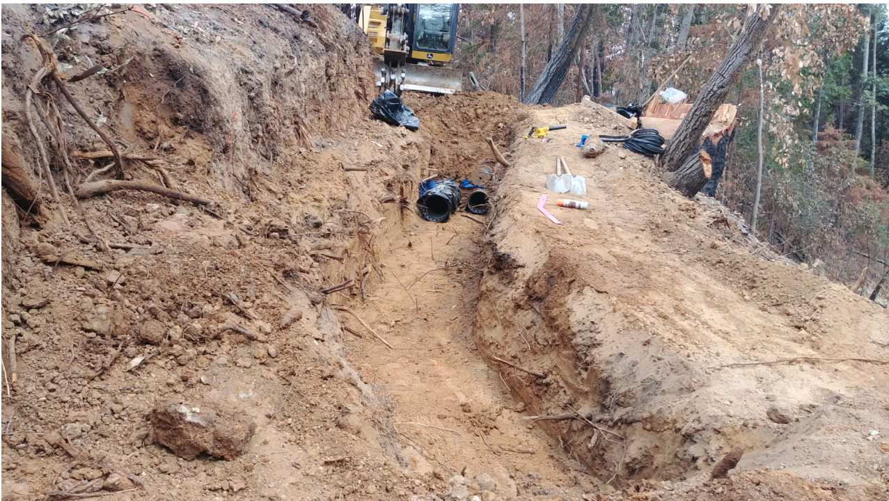
Figure 4: Little Lyon DIP installation
