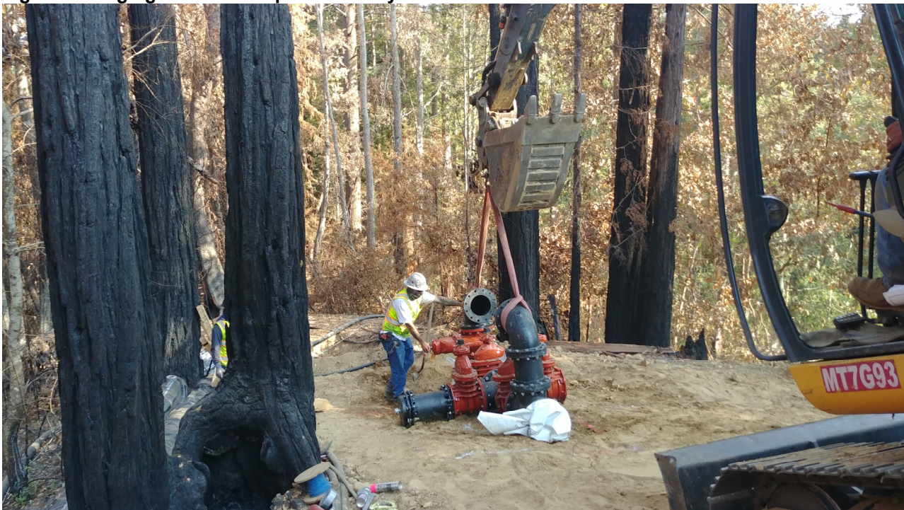
Figure 2: Moving cross and bypass assembly to installation location
