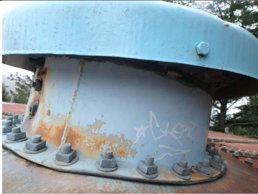
Structural - Roof Structure Roof Vent
