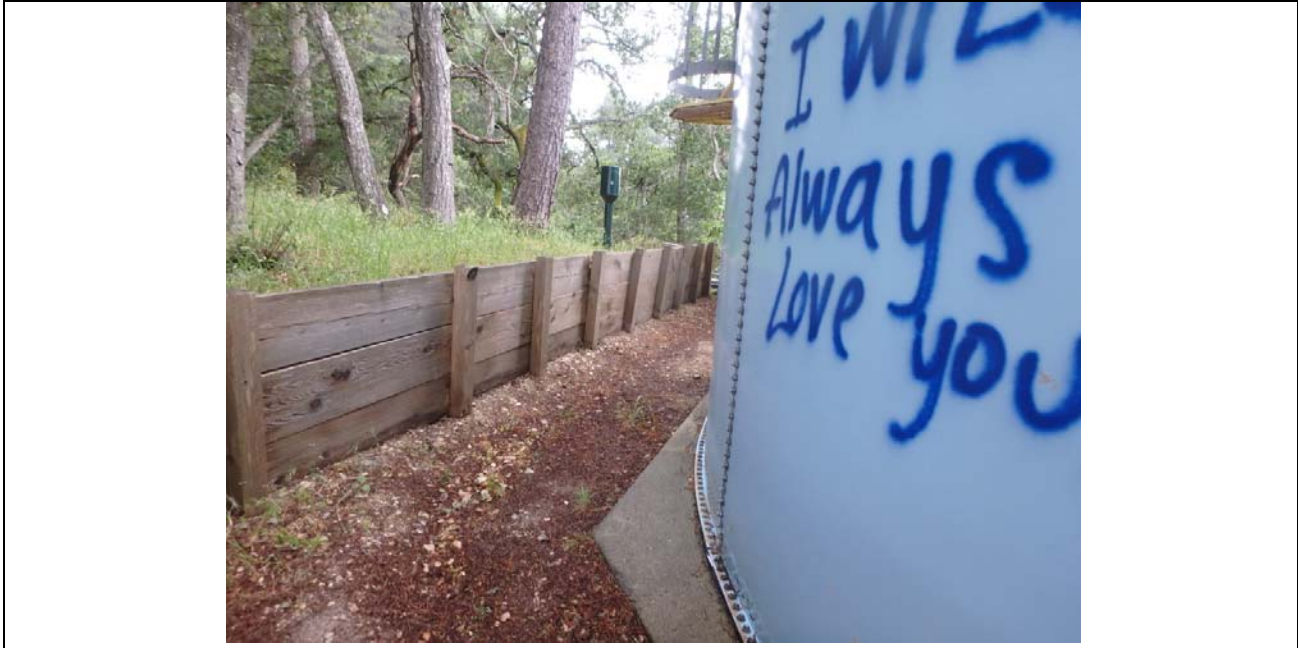
Exterior Coatings Example of graffiti on sidewall.
