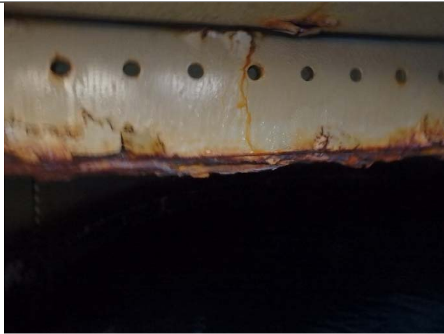
Coating failure and corrosion at the connection point.
