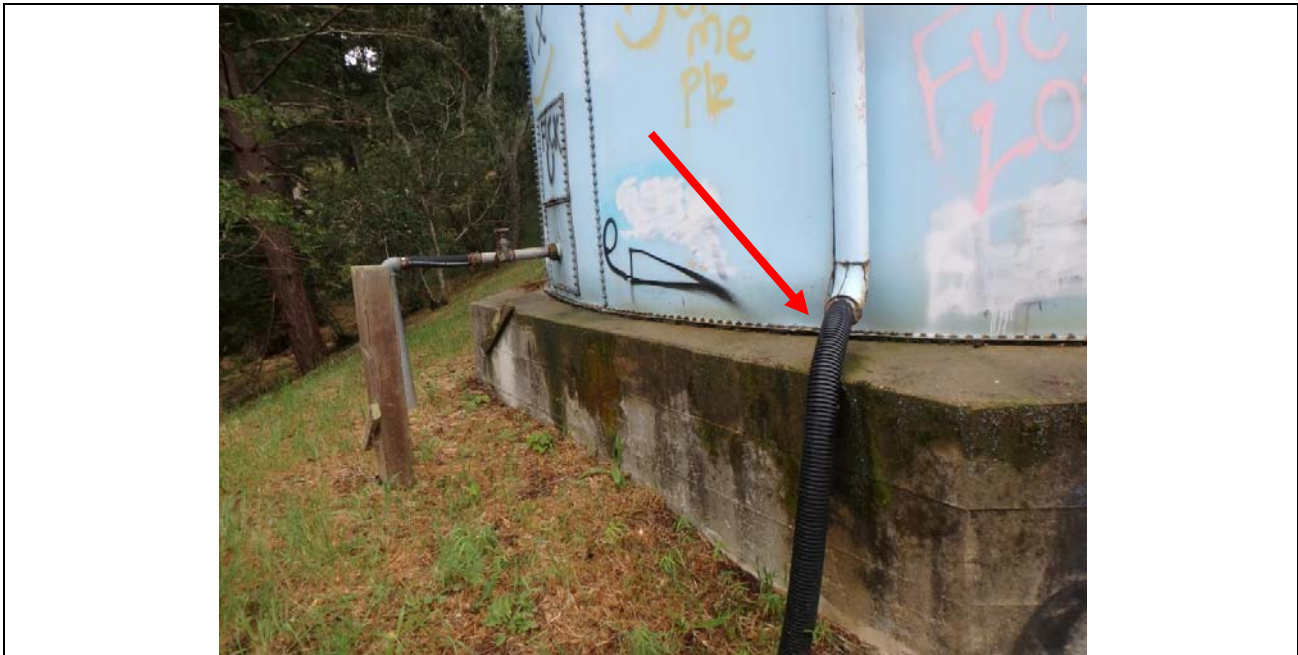
Overflow No air gap.
