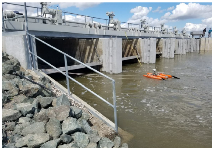
Discharge measurements at the upgraded Wallace Weir Fish Rescue Facility.
