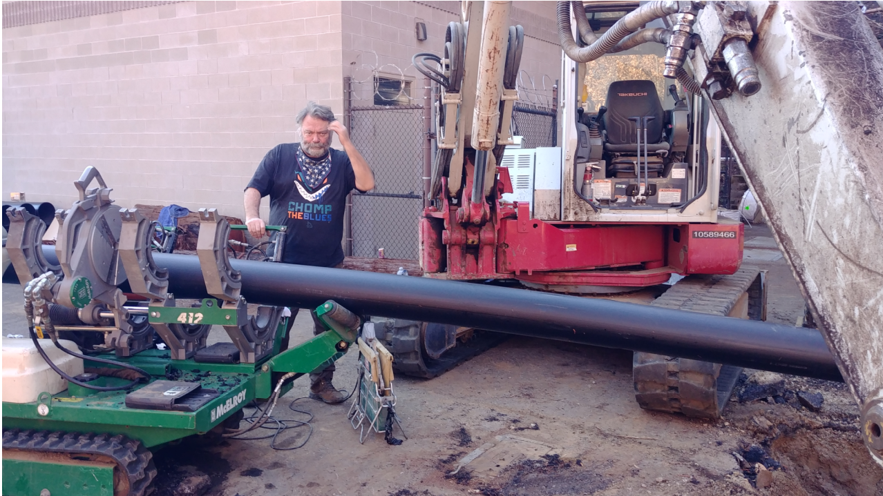
Figure 1: Fusing 8" HDPE for 5-Mile Pipeline
