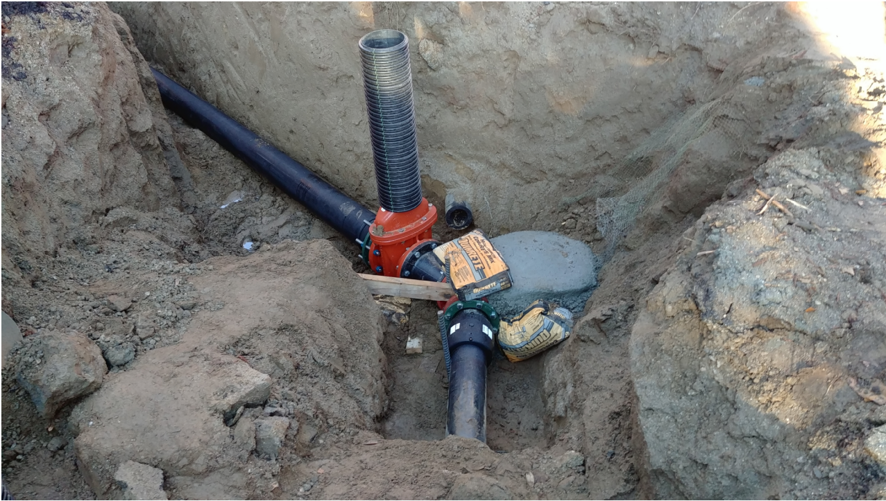
Figure 3: Connection to Existing 8" HDPE 5-Mile Pipeline
