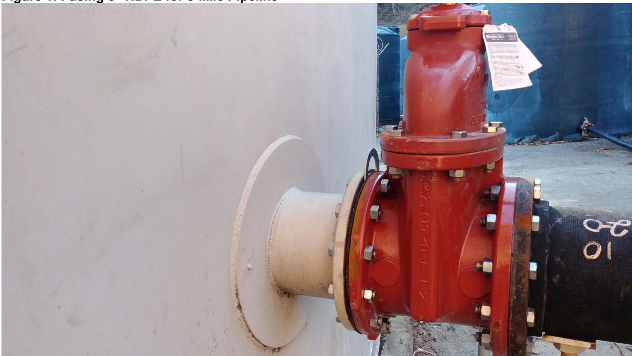
Figure 2: Zone Connection at Little Lyon with Test Plate
