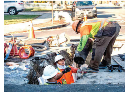
Maintaining the City's infrastructure includes repairing or replacing water mains due to age or condition.
