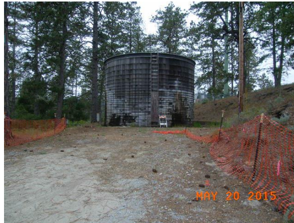
Figure 6D. View of existing Probation Tank, looking northwesterly.
