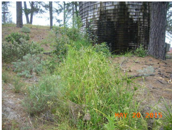
Figure 6F. View of man-made swale that receives water from leaking water tank.
