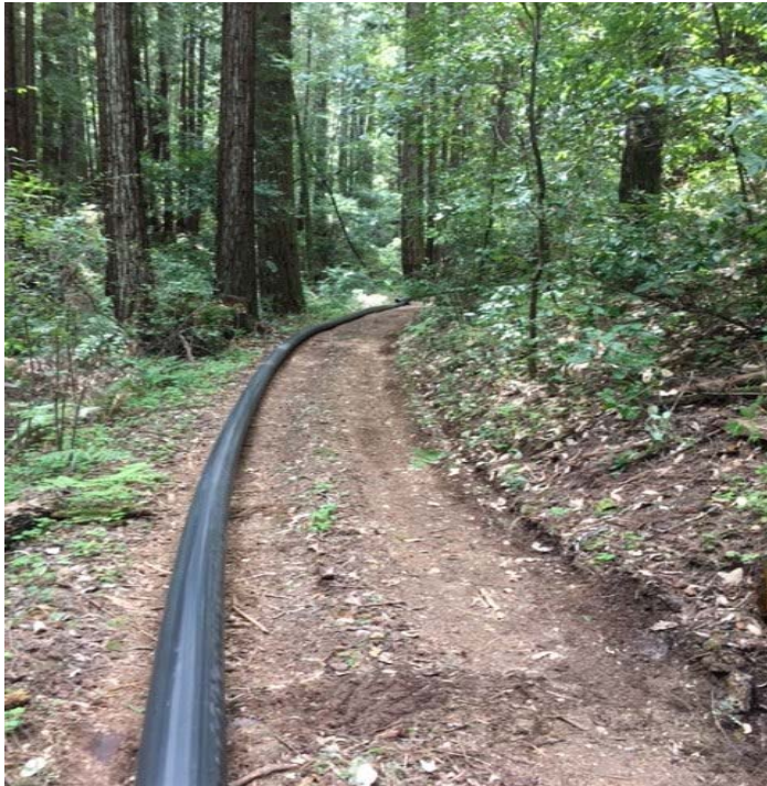
Temporary pipe in roadway
