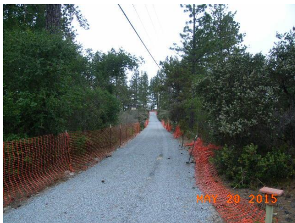
Figure 6C. View of paved access road; existing tank in background amid trees, looking northwesterly.
