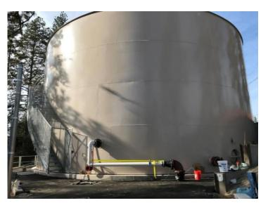
**Project Description:** Construction of a new 500,000-gallon welded steel water storage tank in the Probation Zone. The project included but was not limited to temporary water storage for customers, new water tank, SCADA control, fencing, and environmental permitting.
