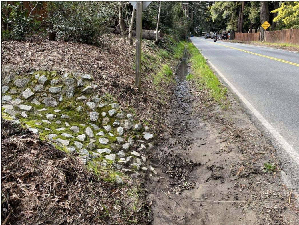
**Photo 2. Unvegetated roadside drainage ditch northwest of Boulder Brook Drive
