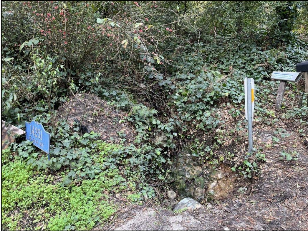
**Photo 3. Incised drainage channel and culvert southeast of Chipmunk Hollow Rd
