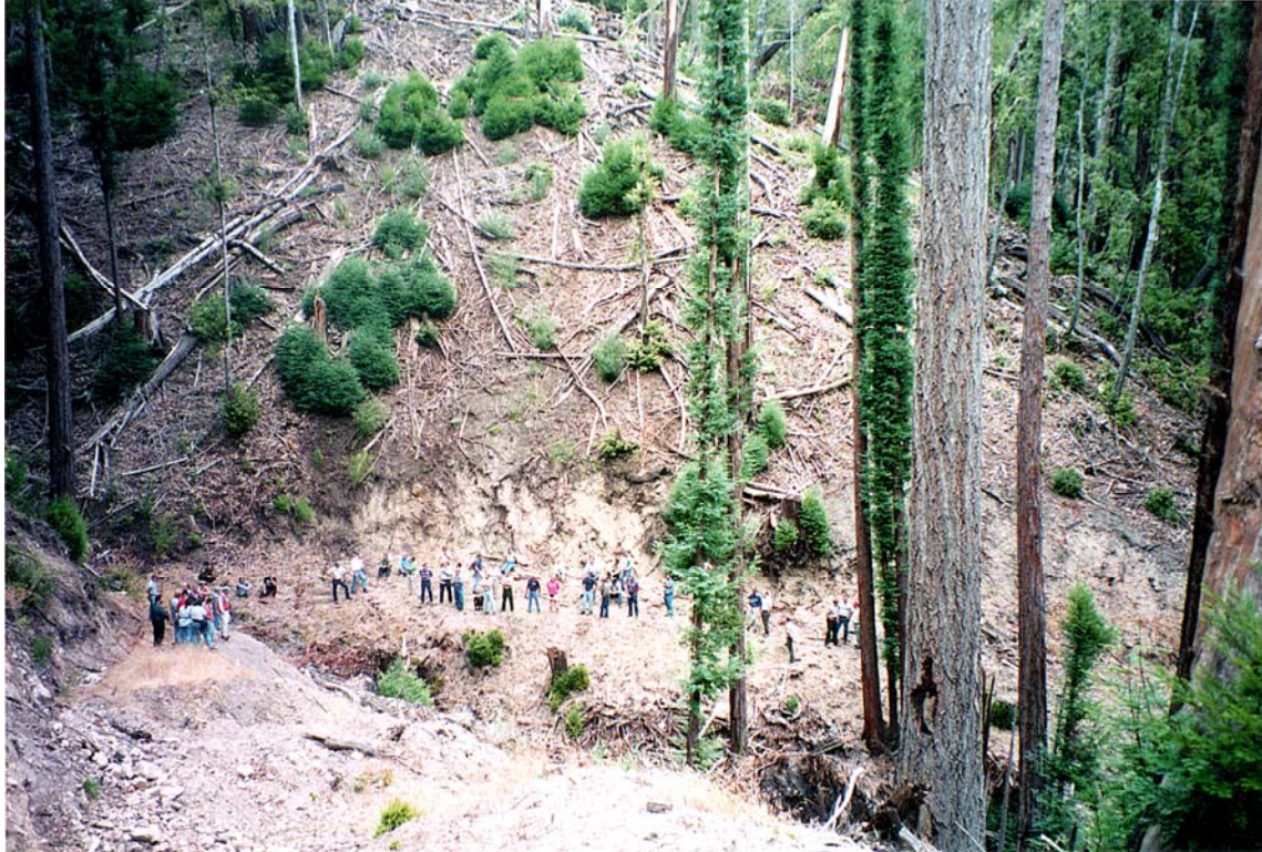
Figure 4-15. Logging road-cut failure on Fritch Creek
