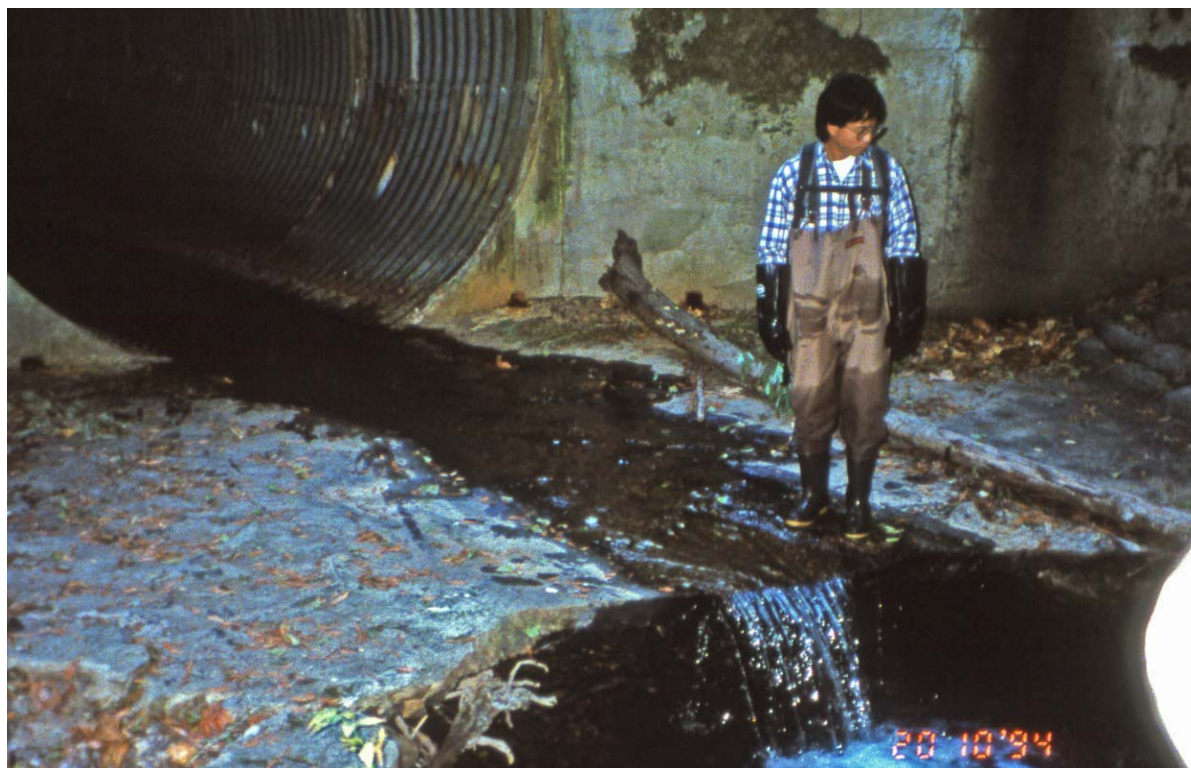
Figure A.24. Concrete apron at the Highway 9 culvert
