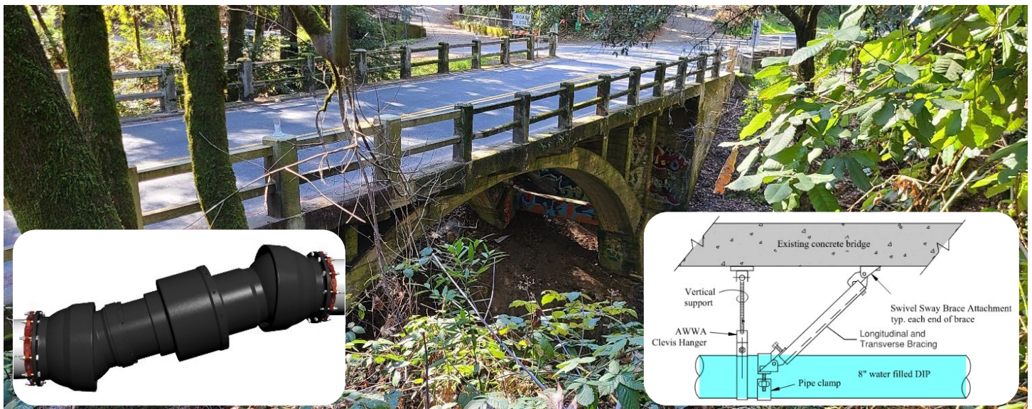
Figure 2 – Water Main Bridge Crossing with Overhang Pipe Supports
