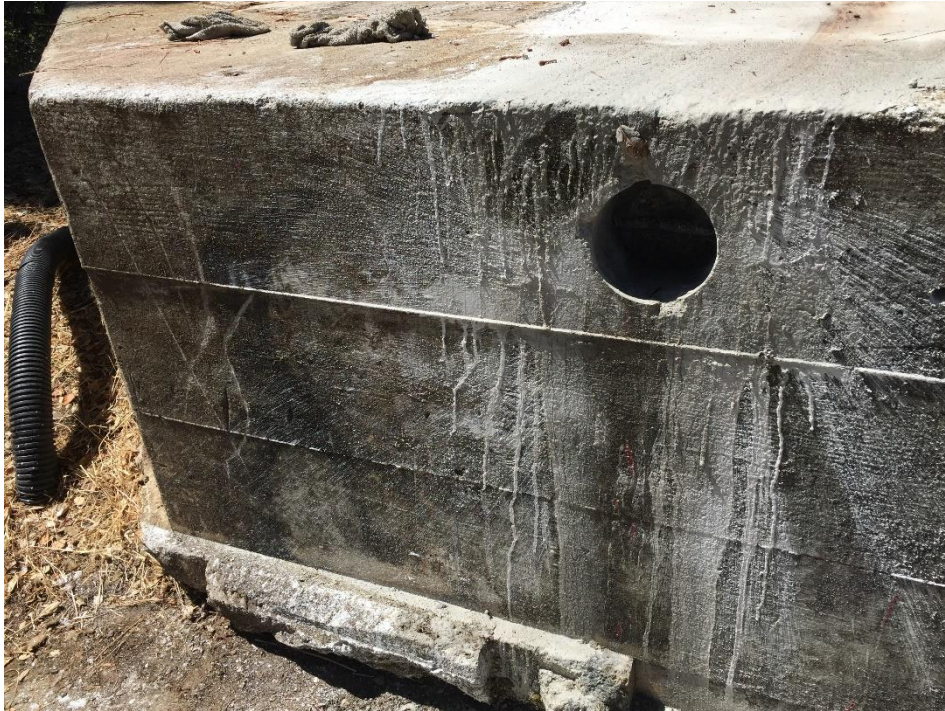
Photograph 3. Core #1 drilled through vertical side of the foundation to expose reinforcement.
