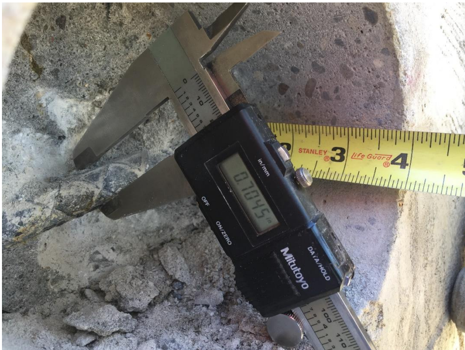
Photograph 4. The rebar at Core #1 was 0.70 inch in diameter and placed 3.75 inches from the vertical side and about 7-inches from the top of the foundation.
