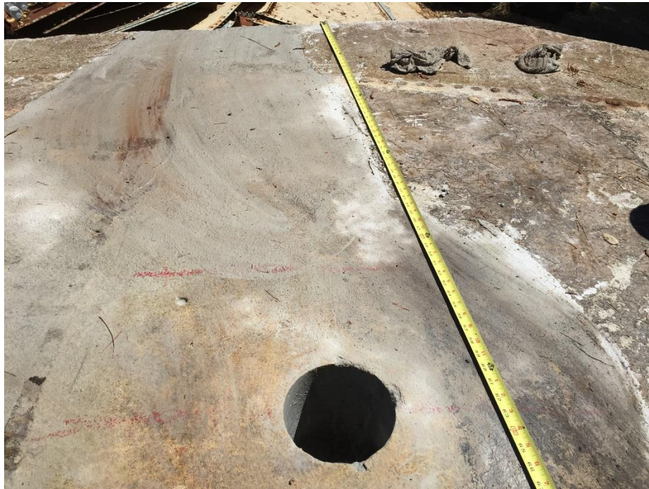
Photograph 5. Core #2 from top of the slab.
