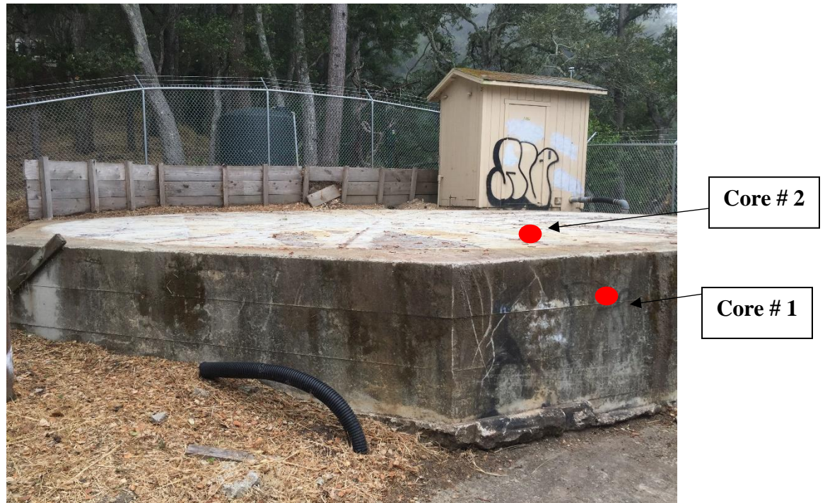
Photograph 1. An overview of the foundation showing core locations.
