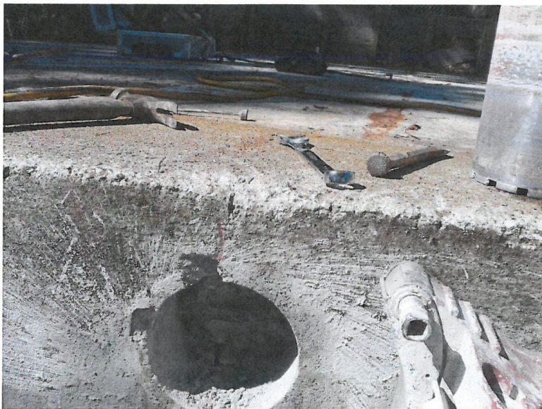
Figure 4 Side Wall Core
