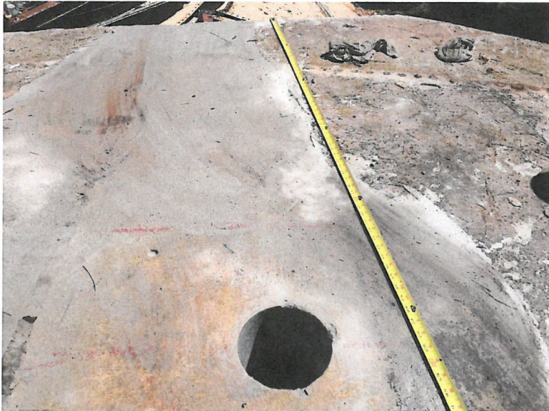
Figure 3 Slab Core
