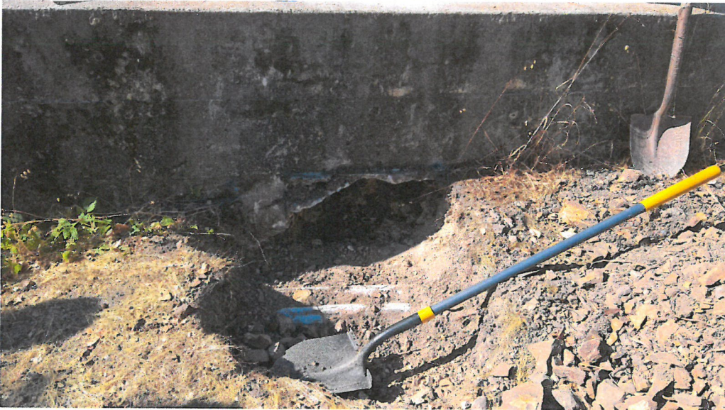
Figure 2 Foundation Excavation
