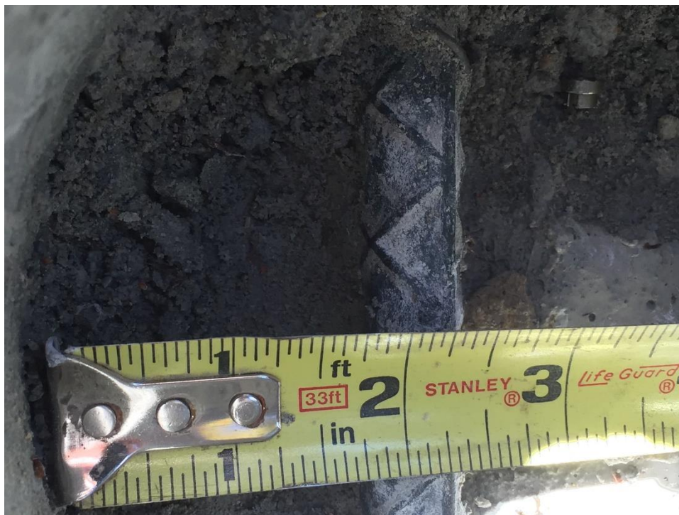
Photograph 6. The rebar at Core #2 was 5/8-inch in diameter and placed 7-inches from the top of the foundation.
