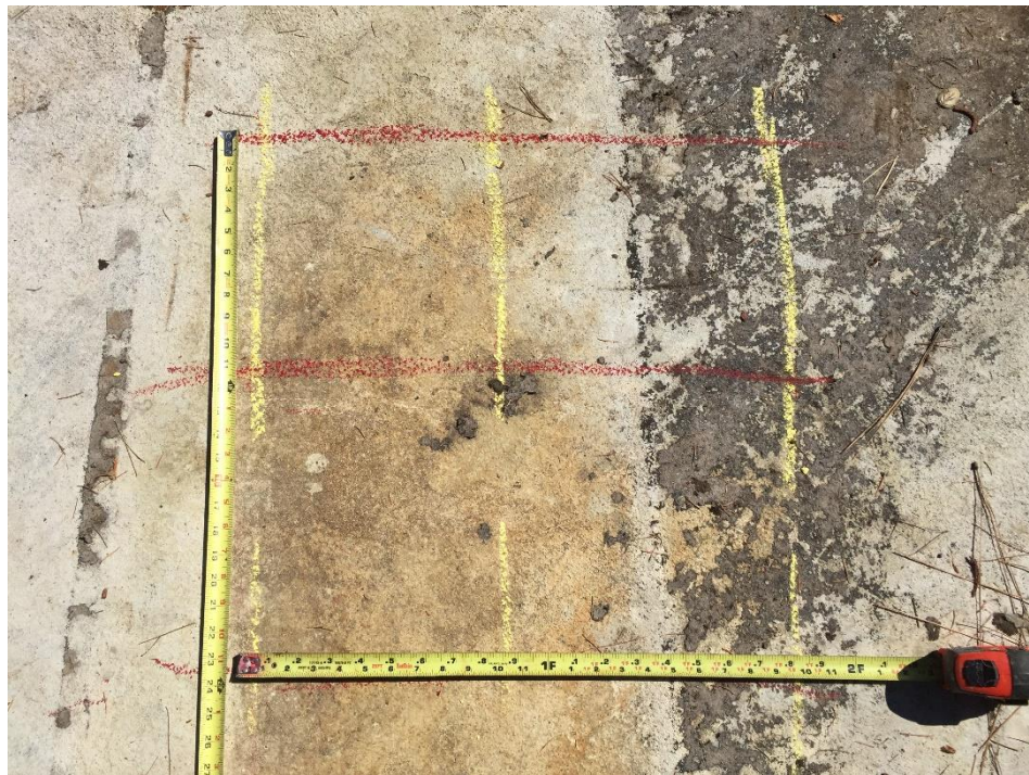
Photograph 2. The radar survey results were marked on top of the foundation. The reinforcement was placed at about 12 inches on center in both directions.
