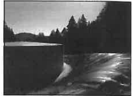
Plastic secures the hillside above the San Lorenzo Valley Water District's 3.5-million gallon storage tank in Boulder Creek.
